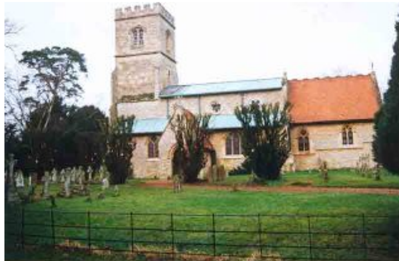
View from the south
