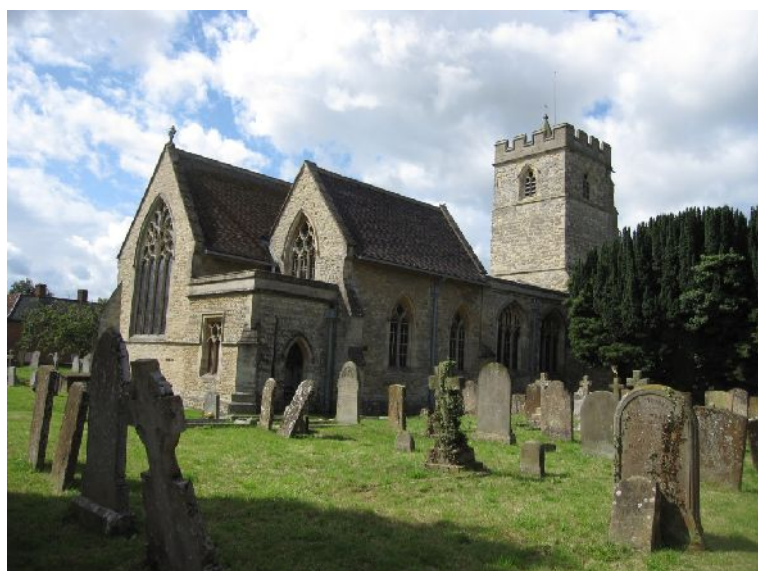
View from north-east
