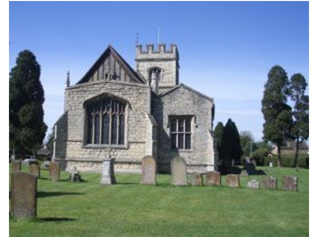
East end of church
