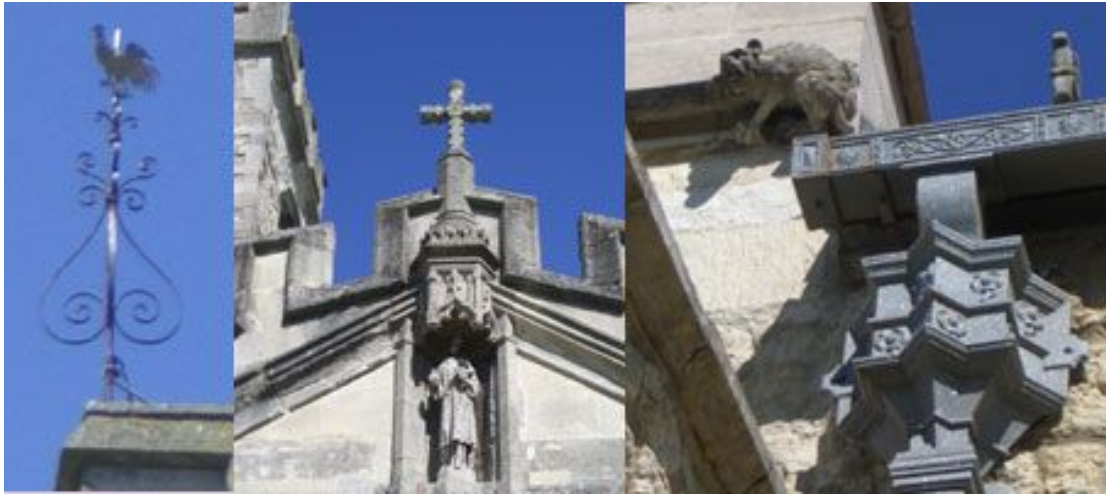
Weathervane and roof detail
