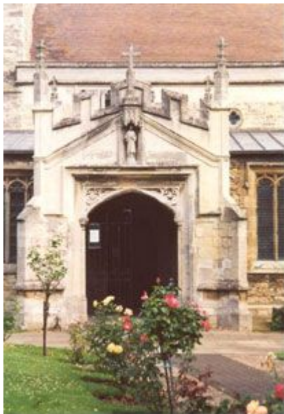
Porch on the south wall
